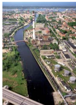
The chimney of SC Klaipeda Energy
