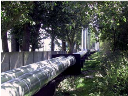
The heat is being delivered through a network of pre-insulated pipelines
